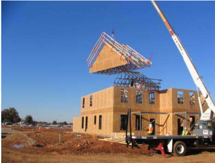
Pre-installed fall protection
