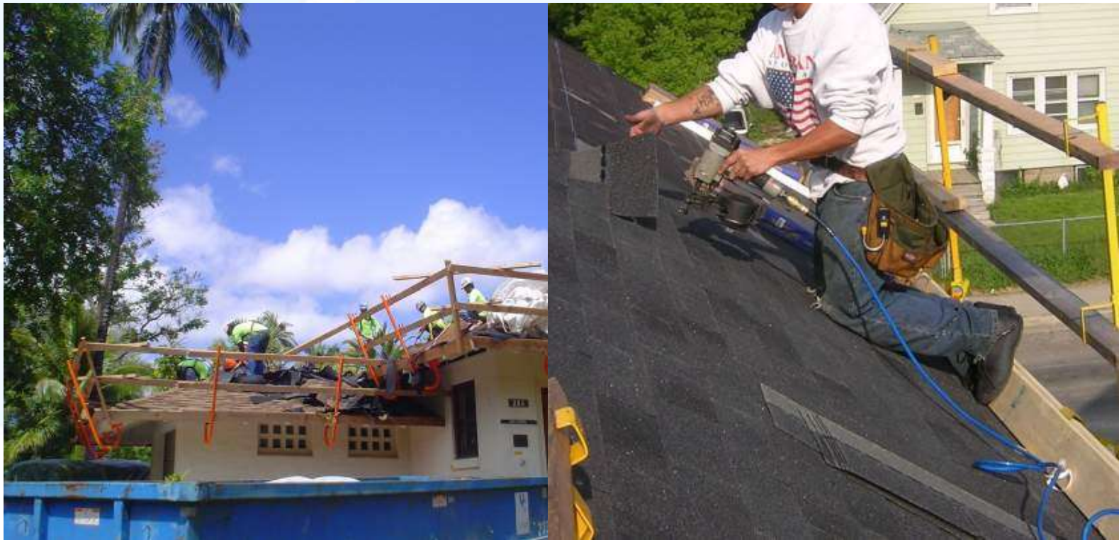
Guardrails in place during re-roofing activities.
