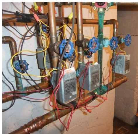
Zone valves: A separate thermostat controls each zone valve. When a thermostat calls for heat, the boiler fires and the zone valve opens.
