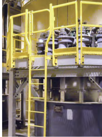
Raised platform with protected guardrail.
