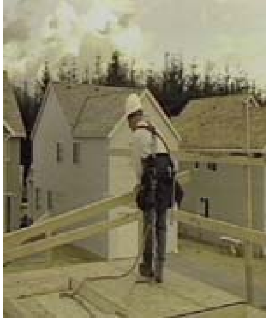
Figure 27 - Worker installing guardrails.
