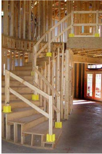
Figure 33 - Wooden guardrail system for a stairway.
