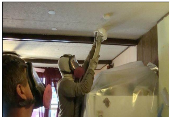
Installing insulation through the ceiling: The technician pushes the fill tube into the cavity and out near the edge of the roof. The holes are drilled in a straight line for aesthetics.
