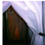
Full containment. (photo courtesy of Terry Brennan)
