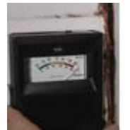
Moisture meter, showing high moisture content in gypsum board behind tile. (photo courtesy of Terry Brennan)
