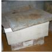
Mold growth on fiberboard shelf (left) and on cardboard boxes (right) due to high humidity. Water is condensing from the basement air, which is at approximately 90% relative humidity (RH). (photo courtesy of Terry Brennan)
