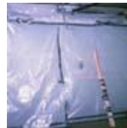
Full containment on a large job. (photo courtesy of Terry Brennan)
