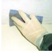
Damp wiping surfaces with water and a small amount of detergent. (photo courtesy of Terry Brennan)
