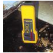
Measuring moisture levels of a sub floor. (photo courtesy of Terry Brennan)
