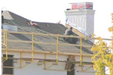
Figure 10 - An exterior bracket scaffold with guardrails being used to protect workers while weatherproofing.
