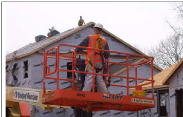
Figure 31 - Worker positioning an aerial lift.
