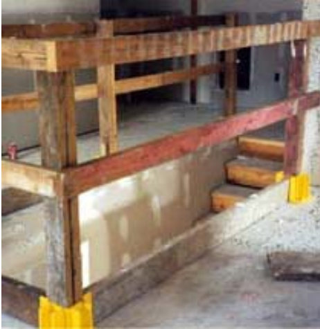
Figures 21 & 22 - Examples of guardrails installed around floor openings.
