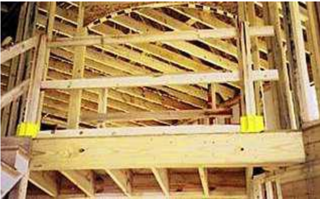
A landing protected by a wooden guardrail system with a toeboard.
