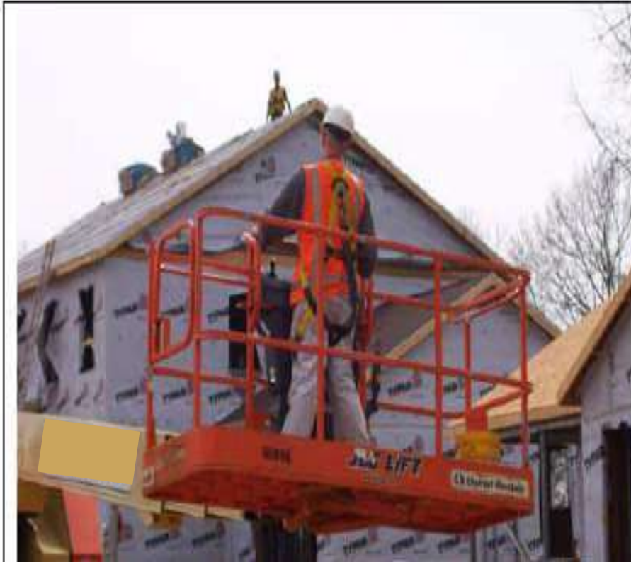
Extensible Boom Aerial Lift
