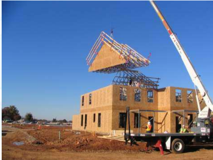
Pre-installed fall protection
