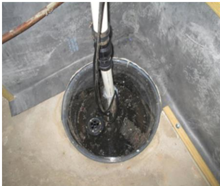
Sump crotch – clear cover-sealed
