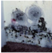
Moldy bedroom closet. Water condensed from the air onto the gypsum board. The wall is cool enough for condensation because there is a hole in the insulation and it is cold outdoors. (photo courtesy of Terry Brennan)
