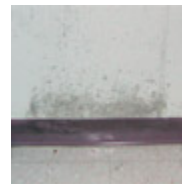
Mold on painted concrete in a school building. Rainwater is wicking directly through the concrete walls, and there is also condensation on the earth-chilled concrete. (The floor is about 3 feet below ground level.) (photo courtesy of Terry Brennan)
