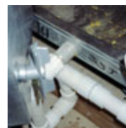
Example of a drain pan beneath a cooling coil that slopes to a drain line and is constructed of stainless steel. (photo courtesy of Terry Brennan)
