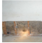
Mold inside a wall. This photo shows an interior wall with the lower portion of the drywall removed on one side; there is mold on the backside of the drywall caused by water leak. (photo courtesy of John Martyny, Ph.D.)
