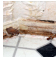
Mushrooms growing at the base of and behind the baseboard below a water leak in a bathroom. The baseboard has been removed; the puckers in the paint are due to water damage. (photo courtesy of John Martyny, Ph.D.)
