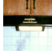
Example of an exhaust hood and fan over a stovetop in a kitchen. An exhaust fan over a range draws heat, moisture, and contaminants out of the house. Range hoods should vent to the outside. (photo courtesy of Terry Brennan)
