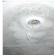
Mold surrounding air conditioning vent in ceiling due to water leak. (photo courtesy of John Martyny, Ph.D.)
