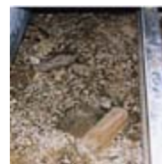
Mineral deposits on the surface of a dirt crawl space caused by chronic water problems. (This is not mold.) (photo courtesy of John Martyny, Ph.D.)
