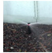
Moisture Issue: A lawn sprinkler is located near the outside wall of a building; the sprinkler sprays the wall directly, and water leaks through wall into the building. Fix: Move the sprinkler away from the building so that water does not wet the walls or collect near the foundation. (photo courtesy of Terry Brennan)
