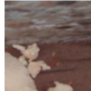
Inside of wall from above, moldy gypsum board, insulation. (photo courtesy of Terry Brennan)
