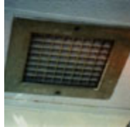
Example of exhaust vent in a bathroom. (photo courtesy of Terry Brennan)
