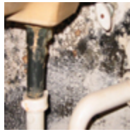
Mold on drywall under leaky sink. (photo courtesy of John Martyny, Ph.D.)
