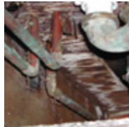
Moisture damage and mold growth under bathtubs. (photo courtesy of Terry Brennan)
