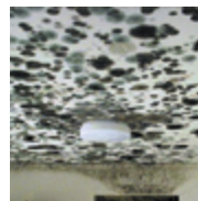
Extensive mold contamination of ceiling and walls. (photo courtesy of Terry Brennan)
