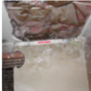
Opening a wall with a utility knife to minimize disturbance to mold in the wall cavity.
