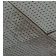
Acoustic ceiling tiles with water damage. (photo courtesy of Terry Brennan)
