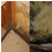
Looking for mold in wall cavities by removing a section of drywall. (photo, John Martyny, Ph.D.)
