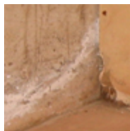
Water in the ground has seeped through the concrete walls of the basement, leaving white mineral deposits on the walls. The water has evaporated into this basement, increasing humidity. Mold is growing in some areas. (photo courtesy of John Martyny, Ph.D.)
