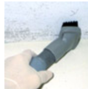
HEPA vacuum. Care is being taken to disturb the mold as little as possible while vacuuming. (photo courtesy of Terry Brennan)
