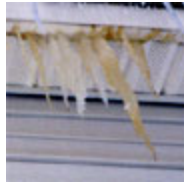
In this case, the icicles result from warm air in the house leaking into an attic without sufficient insulation. (photo courtesy of Terry Brennan)
