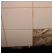
Mold growth under ceramic tiles in a bathroom. (photo courtesy of John Martyny, Ph.D.)
