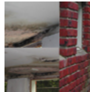
Mold on first floor beneath a through-the-wall air conditioner on the second floor.
